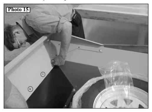
15. Secure all Carriage Bolts by tightening down all Flange nuts. *Photo 16*
